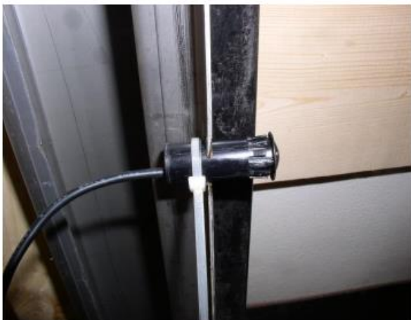
Push Photo cell through hole
