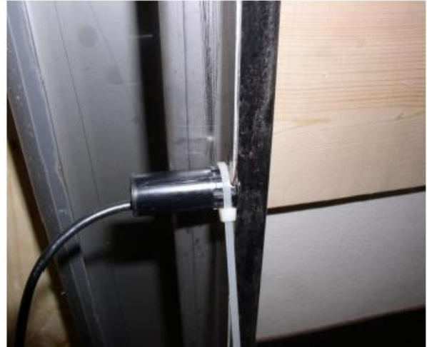
Gently slide tie wrap over retainers of Photo cell
