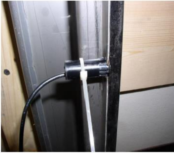
Install tie wrap snug around the barrel of Photo the cell
