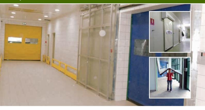
Dynamicroll Food High-speed doors are self-repairing, meaning that if the door curtain comes out of their guides (for example, in the event of impact with a forklift) the system will automatically reset the curtain back into the guide on the next close cycle.
