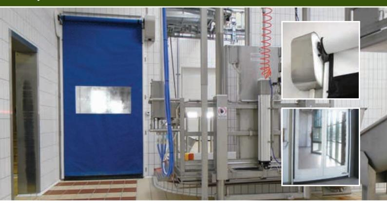
Dynamicroll PE High-speed doors are self-repairing, meaning that if the door curtain comes out of their guides (for example, in the event of impact with a forklift) the system will automatically reset the curtain back into the guide on the next close cycle.
