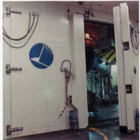
Jamison STC 59 double-swinging jet engine door
